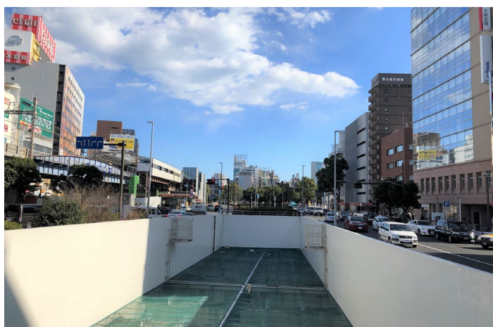
Fig.19 Completed open-cut motorway on the ground level in 2019 Source: own elaboration
