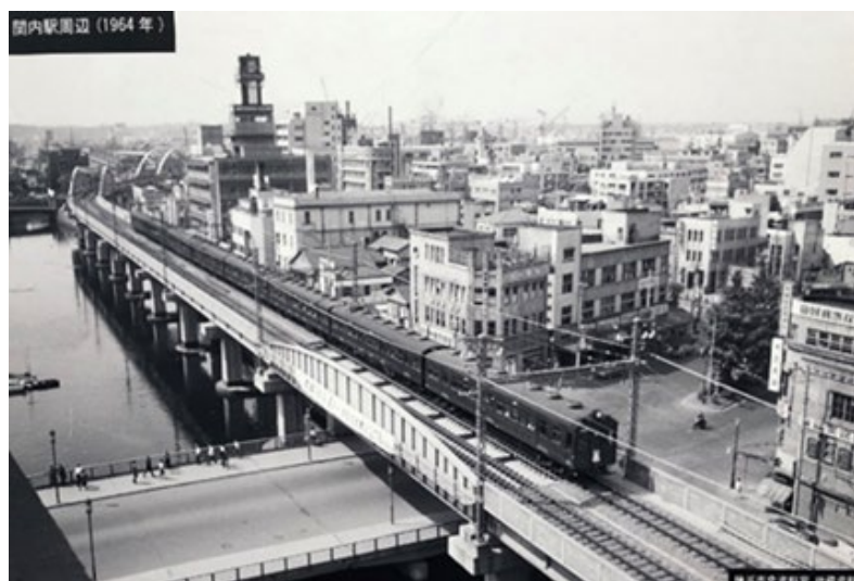
Fig.12 Haohka canal viewing Kannai district on the right. Photo courtesy of the City of Yokohama.
