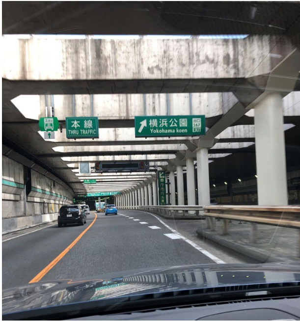
Photo 3 Underground Motorway completed 2018 (Section of open-cut) (Source: own elaboration)
