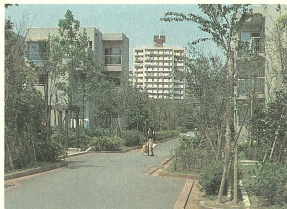
住宅地内の街なみ Townscape in the Residential Housing Area
