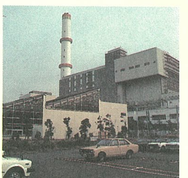
余熱利用施設(港南台) Waste-heat Utilization Facility
