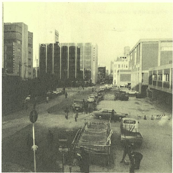
港町くすのき広場完成前 Minato-cho Kusunoki Plaza (before Completion)
