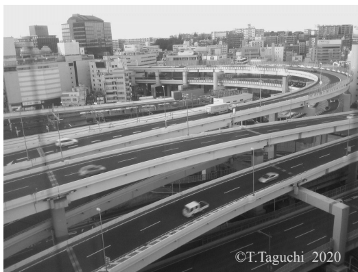
Image of an elevated expressway
